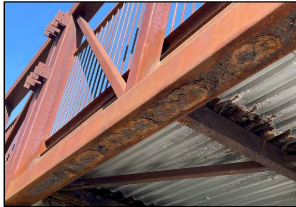
Image 7: Underside of Bottom Chord Delamination
