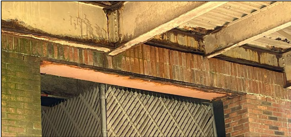
Image 14: North Landing Underside Corrosion
